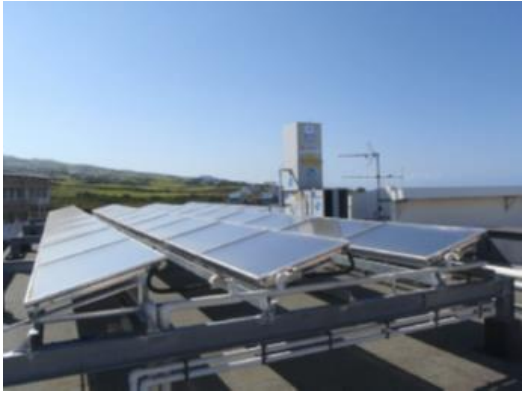
Fig. 1. RAFSOL installation with, on the roof, the solar collector field and the cooling tower (left) and, in the technical room, the absorption chiller and the 2 buffer tanks (right).
